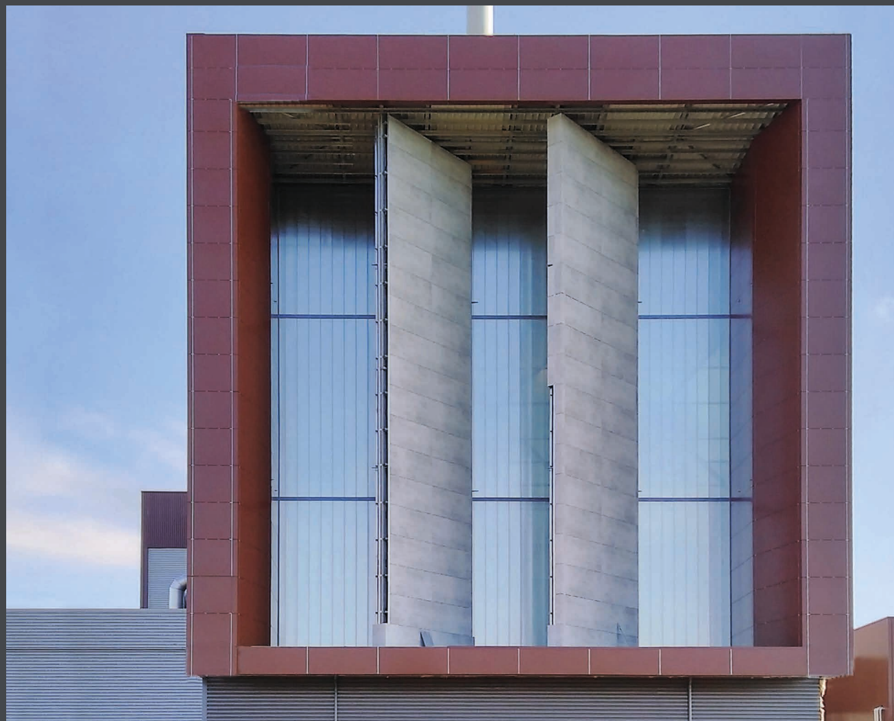
Peterborough Energy-from-Waste facility, Fengate | Material: 250m 2 ALUCOBOND® plus Concrete mat | Building size: W 35 x L 90 x H 34 m Architect: BHP (Birmingham) | Fabricator: Booth Muirie | Installer: KGM
