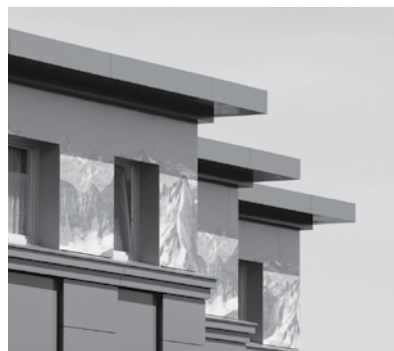
Long-term renewal and maintenance with cost-effective modernisation using ALUCOBOND®: Höxterstraße in Hagen, Germany
