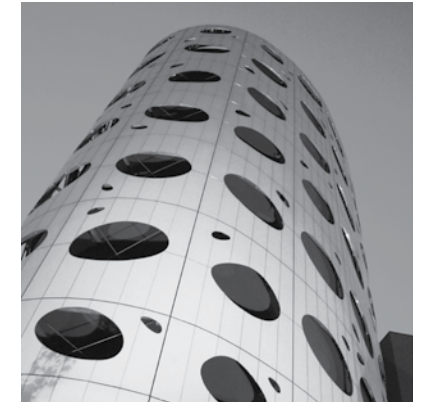
Futuristic architecture with an outer skin made of ALUCOBOND®: the Hotel Lindner Seepark in Klagenfurt, Austria
